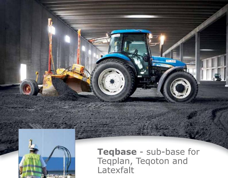
The ideal sub-base for industrial floors! Jointless, large load capacity, quality control.
